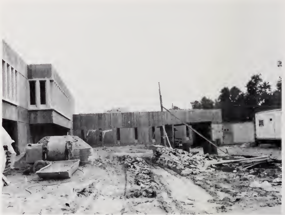
The unfinished Career Center opened this past September.
